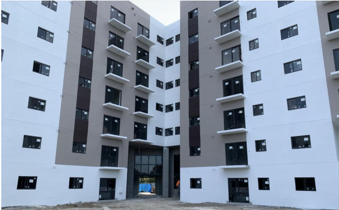
Figure 9 Stadium Towers residential building approximately 92% complete.
