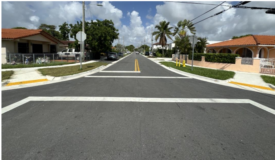
Figure 14 Finished road along SW 24 Terrace
