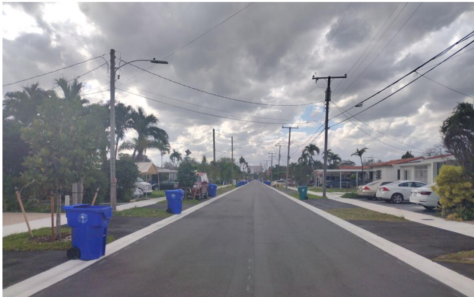
Figure 13 - Finished road along SW 25th Street
