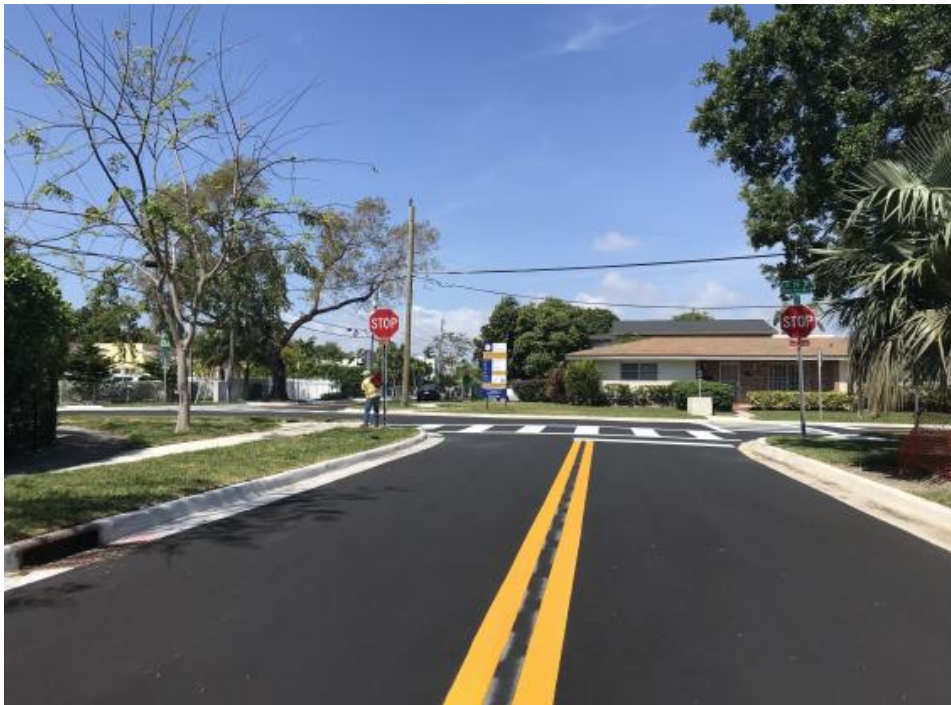
Figure 15 Completed Roadway with pavement markings and curb and gutter.
